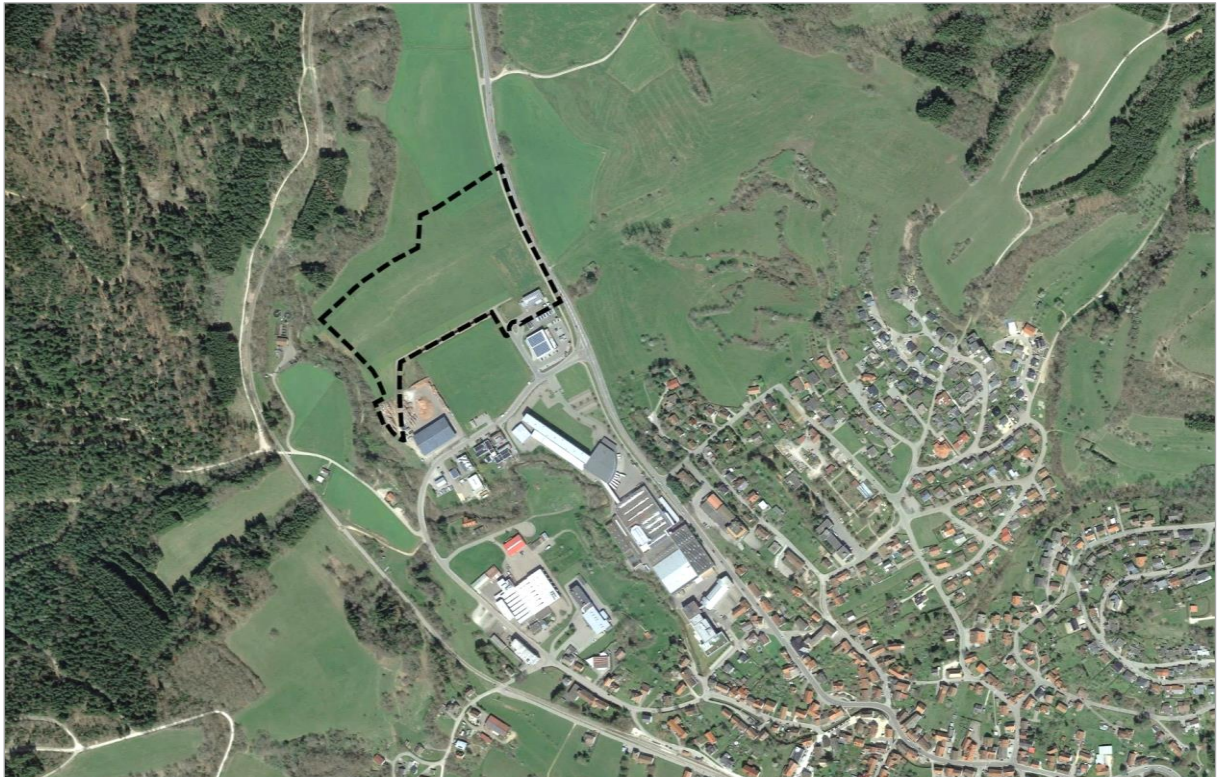
Abb. 7: Bestandsituation – Luftbild (Google Earth)
